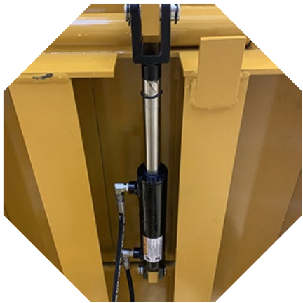
Double action lip cylinder on the lip. Lip rotation by hydraulic force.
